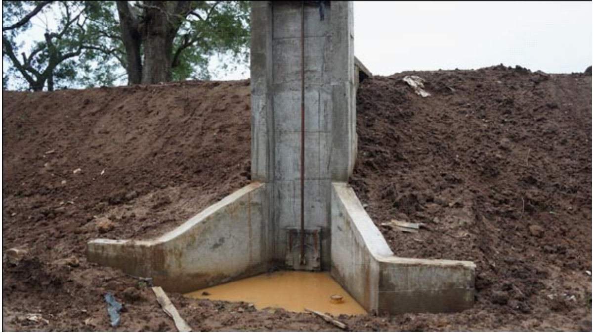
Different looks of agro tank sluice after construction
