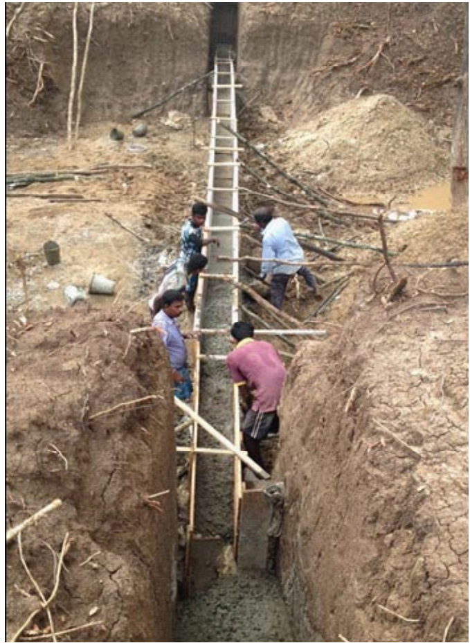
Tank Breach is filled with concrete pilling
